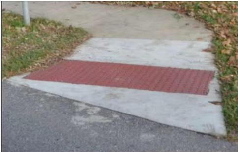
Grade B – Minor Deficiency: The curb ramp shown on the left lacks required turning space.
