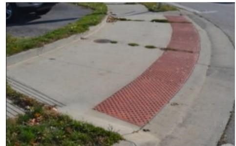
Grade C – Major Deficiency: The curb ramp on the right does not have the required running slope, is overgrown, and the detectable warning is worn out. Curb ramps with no detectable warning automatically receive a grade of C.
